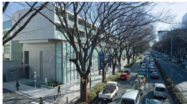
Omotesando Hills complex: a new landmark opened in 2006
